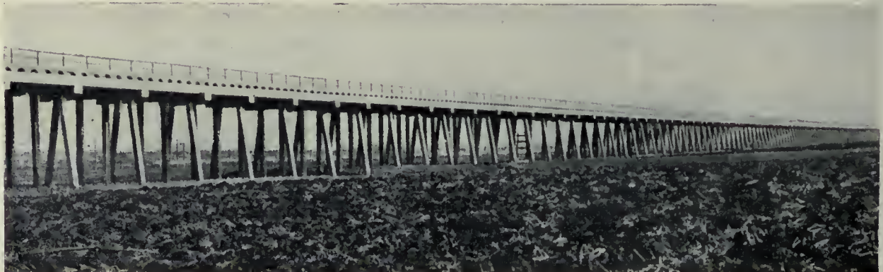
Reinforced concrete highway trestle 3\frac{1}{4} miles long over Yolo By-Pass, California.
